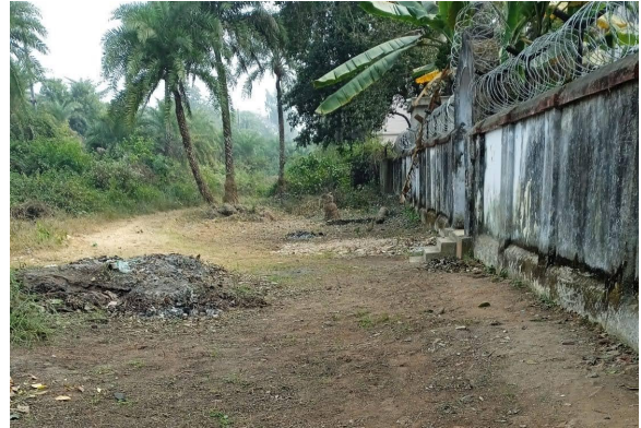
Cleanup of outside perimeter wall
