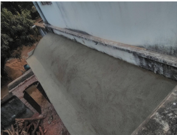
New roof on the east side portico of Shanti Ashram
