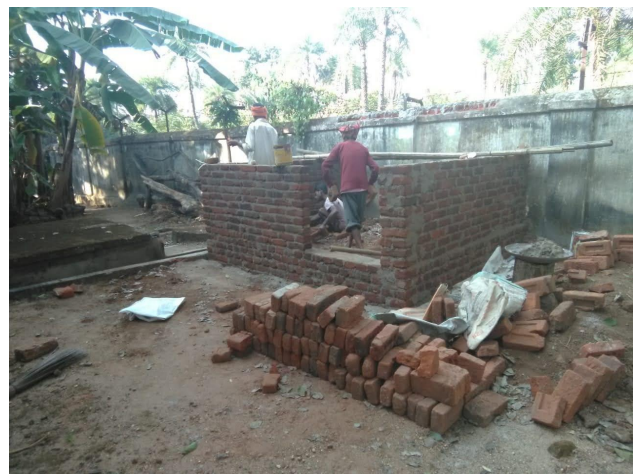
A new guest bathroom with western facilities in construction
