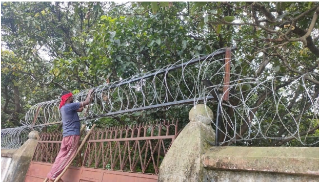
New perimeter fencing being installed.
