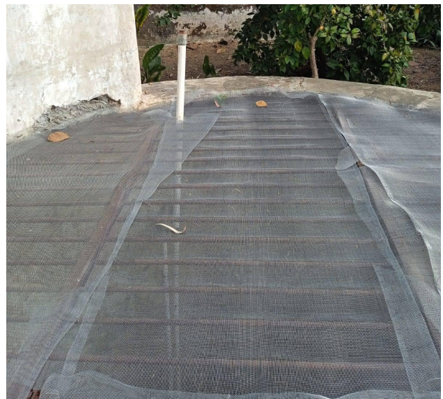
Steel screen over wells
