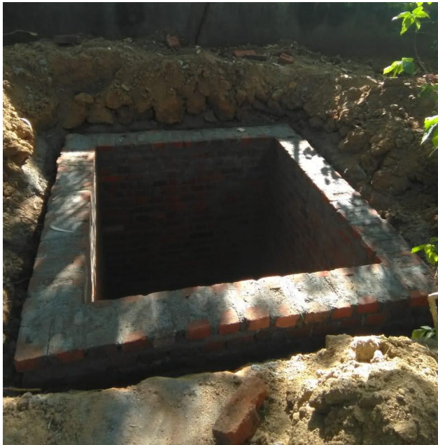
A new underground water tank
